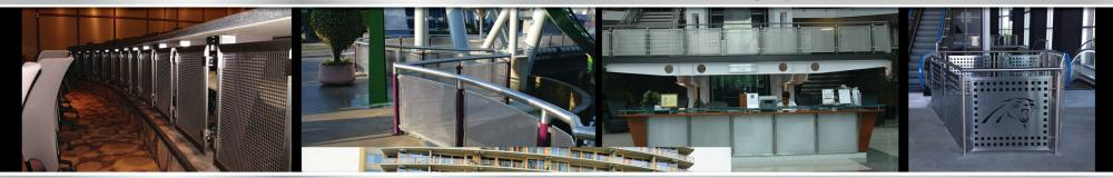
**RAILING STYLE – SILVER SPRINGS** 2 & 3 Line Railing System With Captured Glass Panels.
